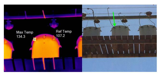
**Comments:** This center transformer has a thermal pattern consistent with a loose or corroded secondary tap connection.
