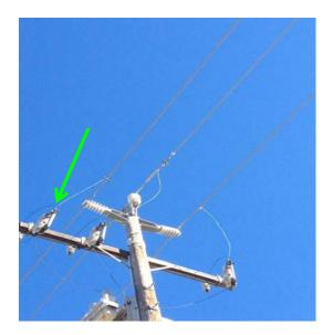
**Comments:** This left fuse has a top connection defect. It has been reported on multiple times and has continued to increase in temperature.
