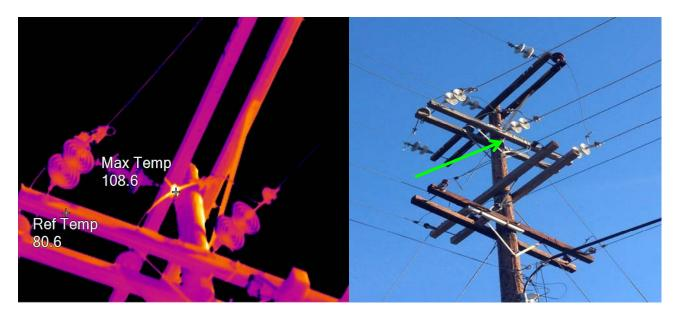
**Comments:** This middle line has a thermal pattern on the clamp connection consistent with excessive resistance. Typically this is a result of a loose or corroded clamp connection.
