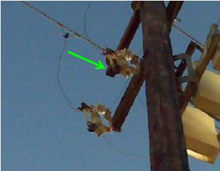
**Comments:** This middle fuse has elevated thermal pattern on the line side B phase connection. It has been reported on multiple times and has continued to elevate in temperature.
