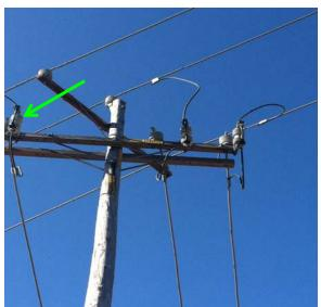
**Comments:** This left fuse has a bottom connection defect. It has been reported on multiple times and has continued to elevate in temperature.
