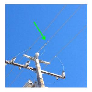
**Comments:** This middle line has a "U" clamp connection that indicates a defective condition resulting in elevated thermal pattern, this appears to be a result of excessive resistance at the mechanical connection. This is a new defect.
